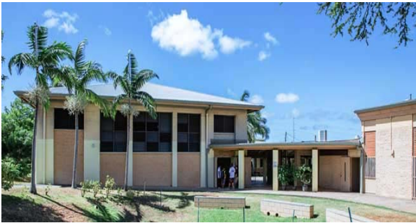
$50,400 Repairs to Exterior Building
